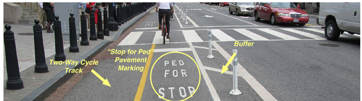
Figure 8. Two-way cycle track near F Street intersection.
