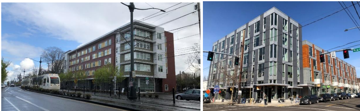
3 4 5 Figure 2: Portland Central TODs, apartments with ground-floor retail (left and right)
