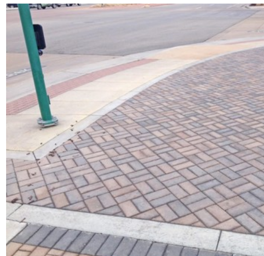
The elevation change of the curb ramp is indicated by a different paving pattern. The orange marked crosswalk design is consistent throughout North Temple (1460 West). Portion of the curb protrudes into the road to assist visually impaired people to navigate the street.
