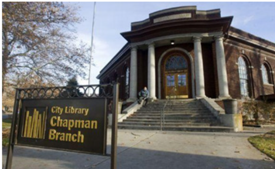
Chapman Branch Library
