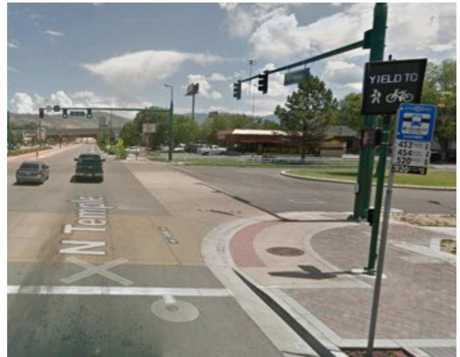
This intersection at 800 West, which experiences a high volume of traffic daily, has marked crosswalks, countdown beacons, LED “Yield to...” signage, traffic signals, buffers, and tactile paving with LOOK pavement markers. Source: Google Maps Street View.
