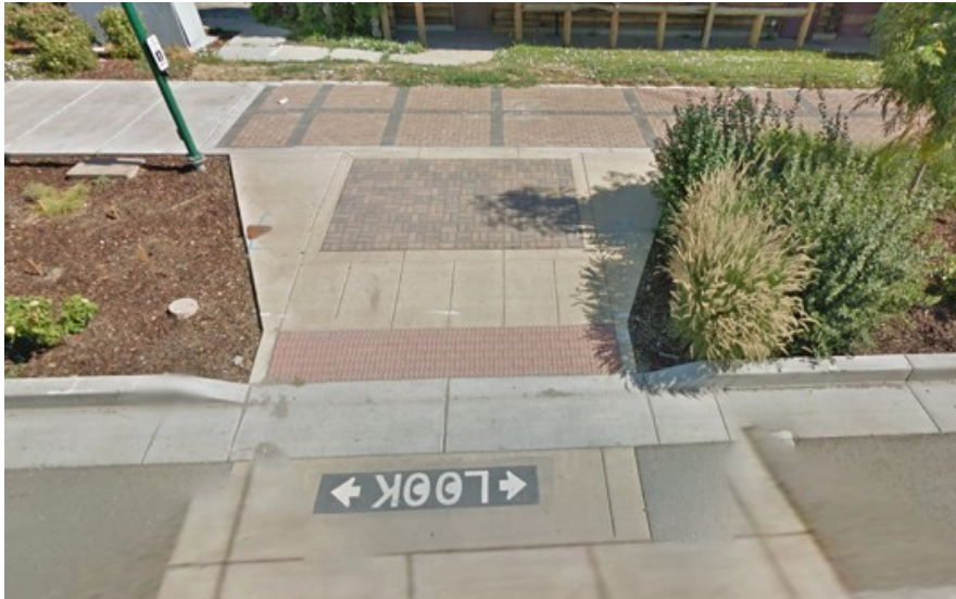
This marked mid road pedestrian crosswalk at 1528 West (Trax Power Station), contains a variety of tactile paving to indicate the elevation changes. In addition, the presence of countdown beacons, a dedicated traffic signal, automobile buffers and LOOK pavement markers. Source: Google Maps Street View.
