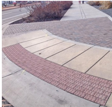
Truncated domes adorn every intersection and crossing along North Temple. Highly visible, tactile paving is used to indicate elevation changes.
