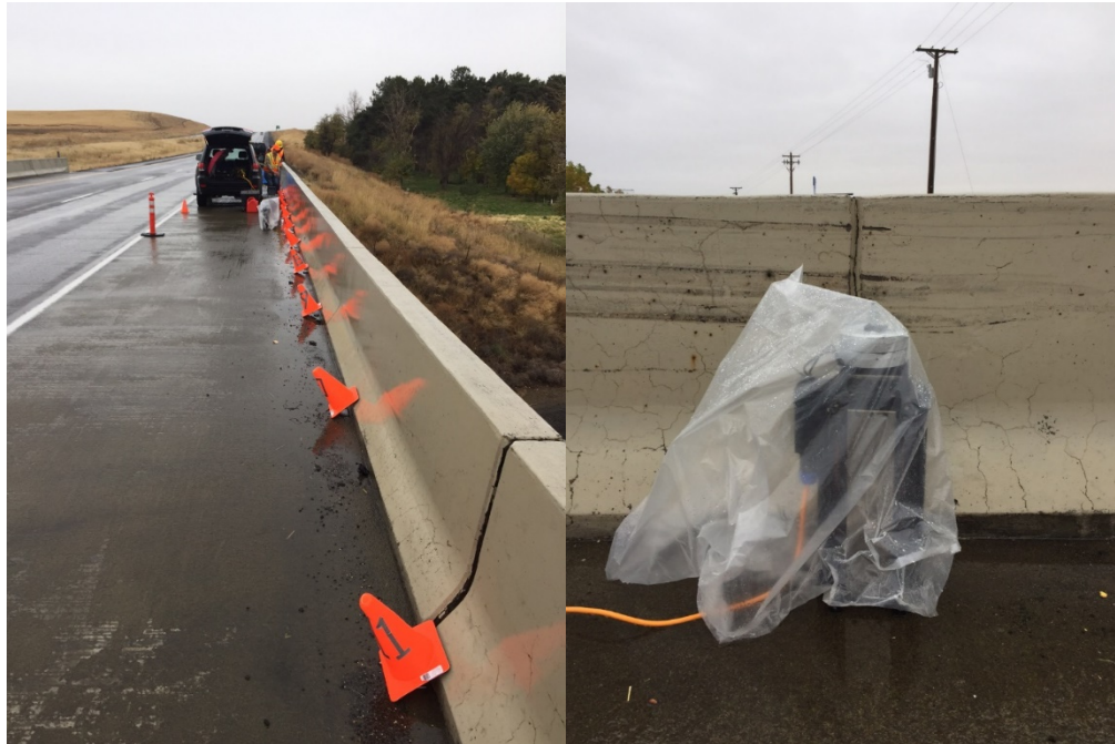
Figure 4.42: Test setup at barrier and protected shaker.
