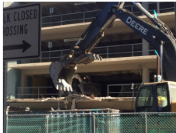
Second floor office demolition
