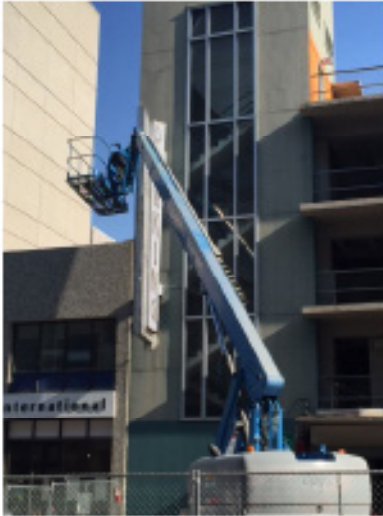
Dismantling of "parking" sign
