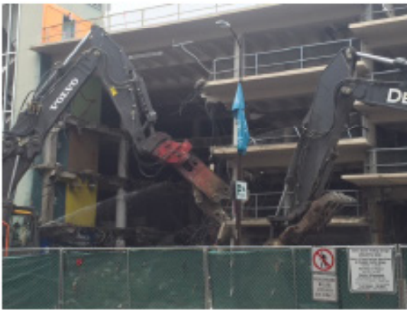
Demolition of Levels 1-3
