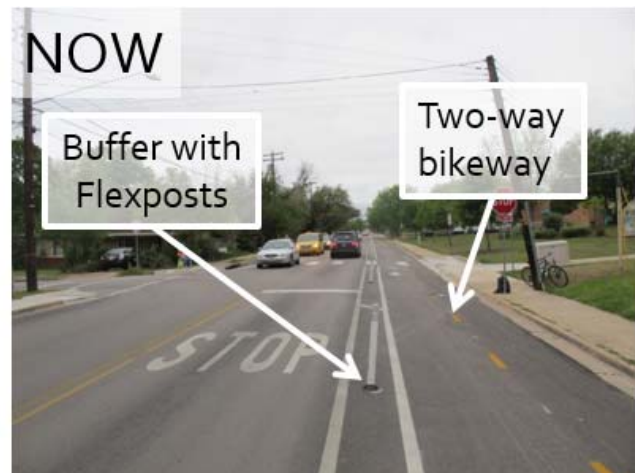
Figure 3-10. Bluebonnet Lane, Austin, TX, Before and After Installation of Protected Bike Lane
