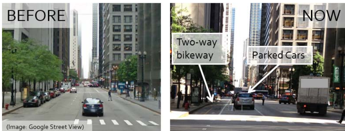
Figure 3-17. Dearborn Street, Chicago, IL, Before and After Installation of Protected Bike Lane
