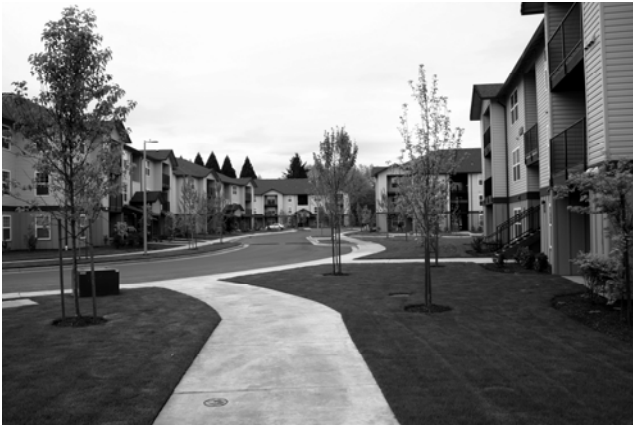
Figure 2: Typical Suburban Multifamily Housing (clockwise from upper left: Eugene, Oregon; Phoenix, Arizona; Sun Prairie, Wisconsin; Pleasanton, California)
